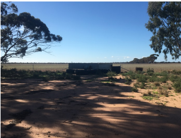
Fencing – Needs Replacing
