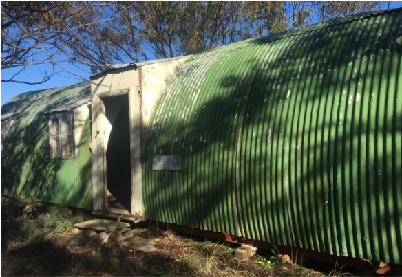
Nissan Hut – Old Clubhouse
