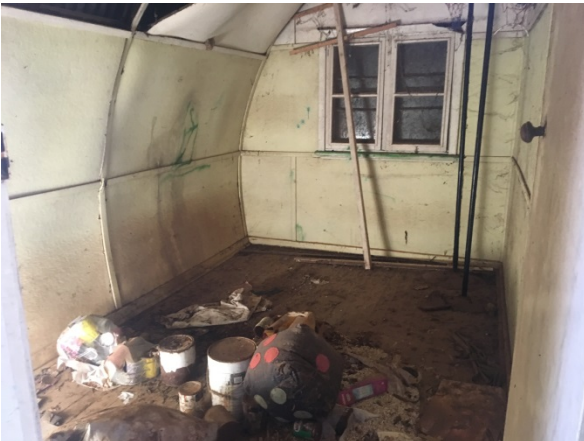
Inside Nissan Hut – Old Clubhouse
