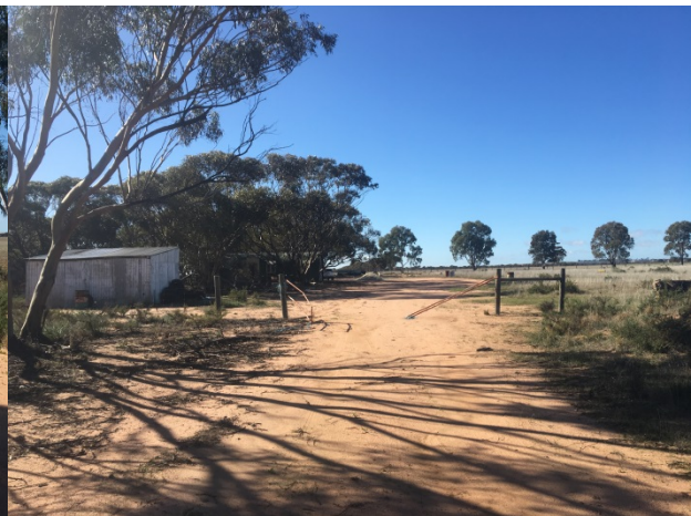
Gate – Needs Replacing
