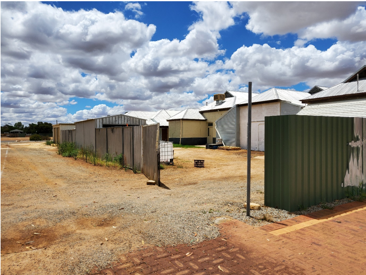
View long western boundary looking from Churchill Street
