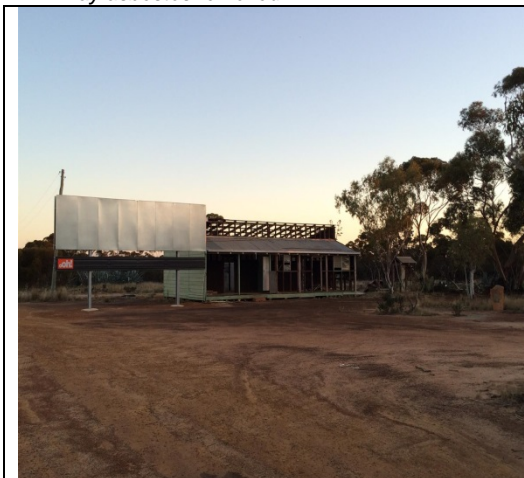
27 th May asbestos removed
