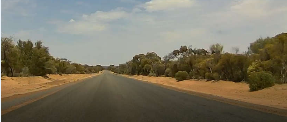
Figure 14: Existing Westonia Road Formation
