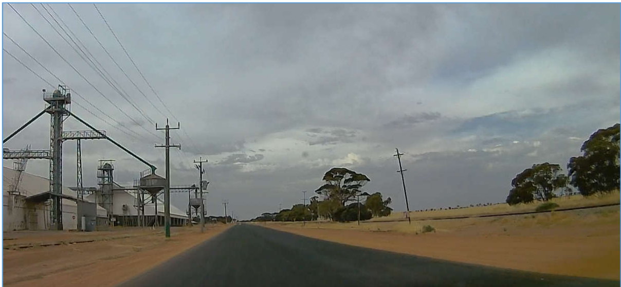
Figure 9: Existing Latham Road Formation – Upgraded Section Adjacent to CBH Grain Facility
