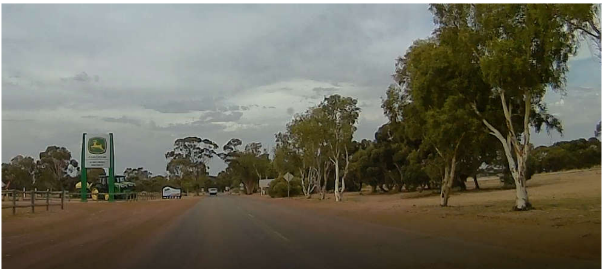
Figure 7: Existing Kondinin – Naremben Road Formation
