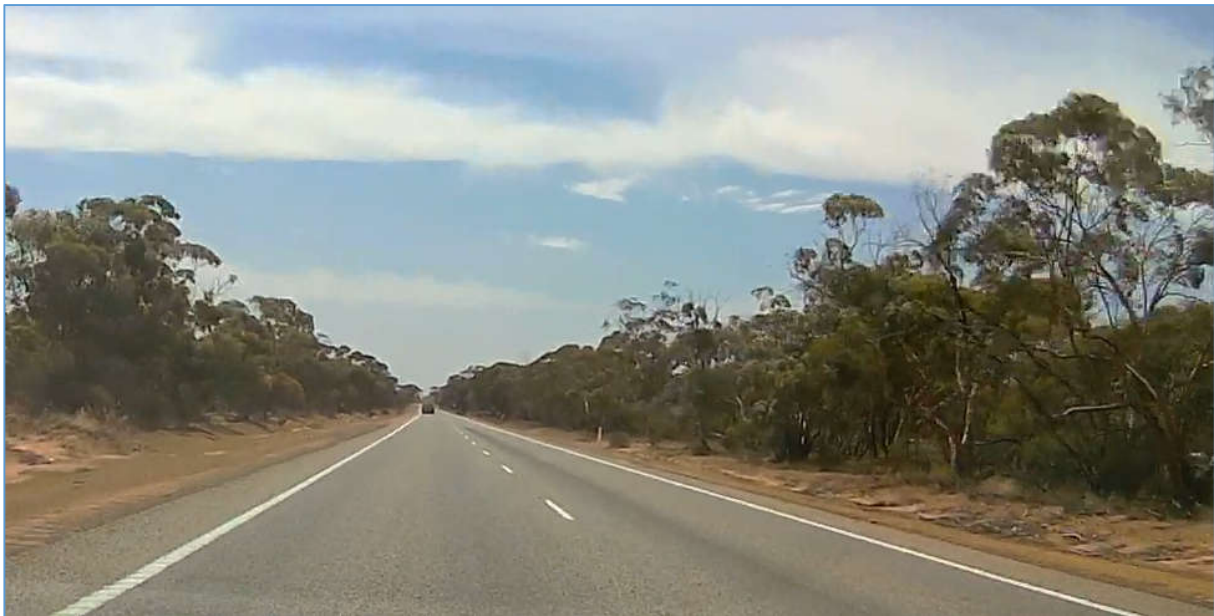
Figure 13: Existing Great Eastern Highway Formation
