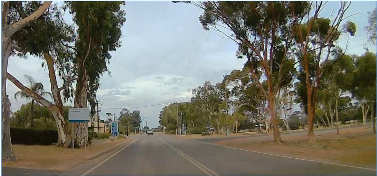
Figure 8: Existing Latham Road Formation – Through Townsite
