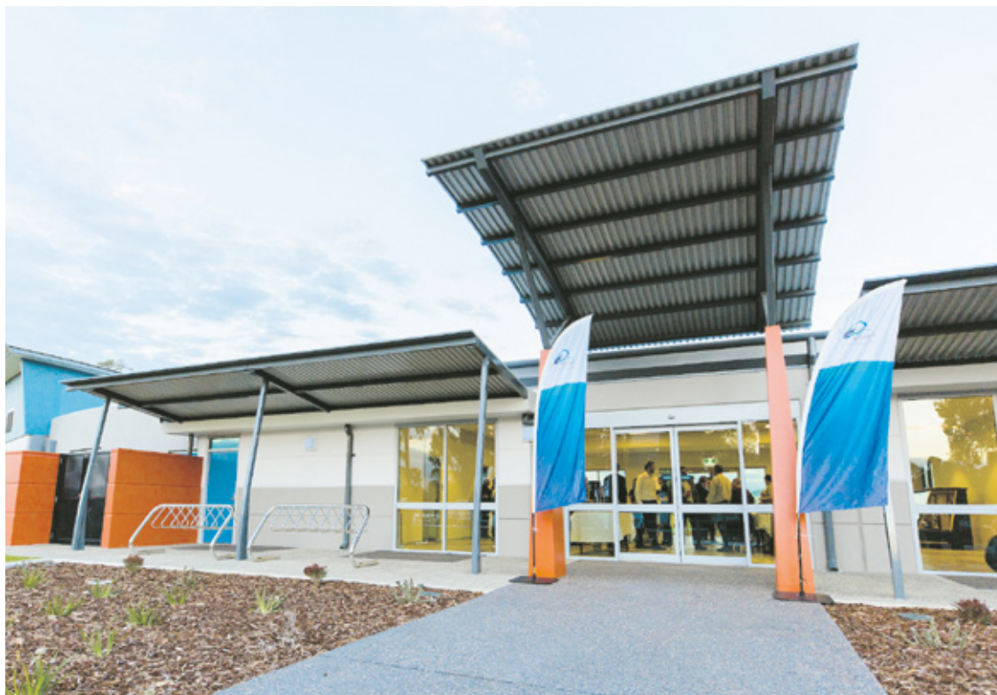
City of Rockingham's new Baldivis South Sporting Pavilion
