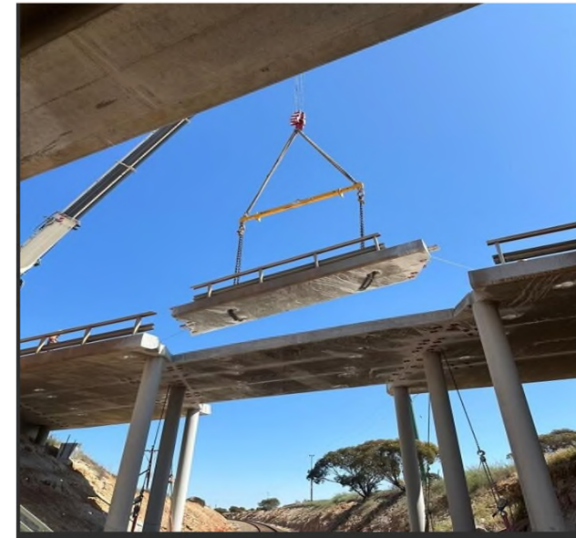
Bridge 629 on Great Eastern Highway
