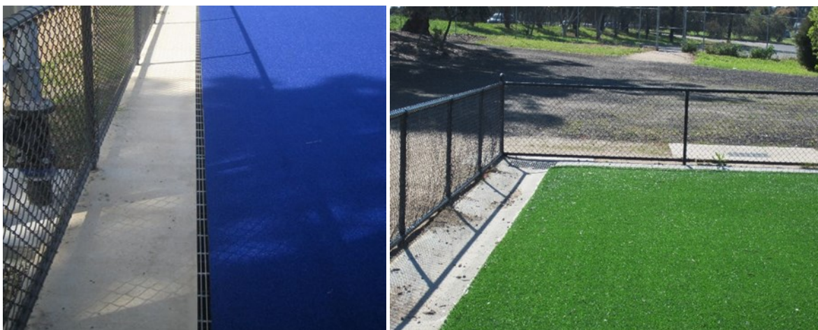
Figure 14: Profiles of spoon drains
