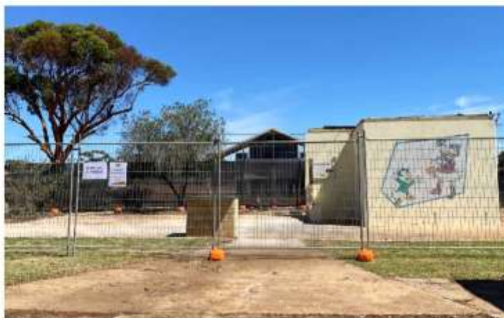
Public Toilet at Apex Park—Demolition commenced
