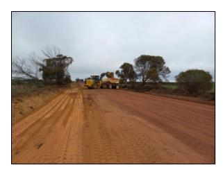
Preliminary works on Coverley Road have been completed in preparation for gravel resheeting between SLK 3.2 and 8.96. This project is funded through the Roads to Recovery program.
