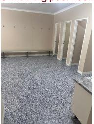
We are pleased to share that the pool building now has an epoxy coating over the floor in the main walkway and all wet areas. The epoxy coating is a substantial aesthetic improvement and offers added safety to pool visitors by significantly reducing the risk of slipping.
